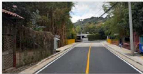
Puente Vehicular RN 105
