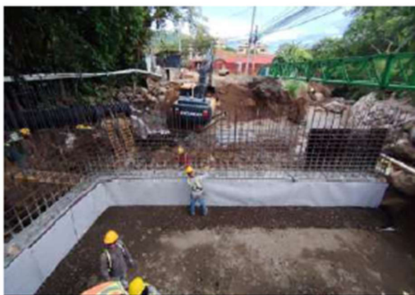
Puente RN 17, Avance 20%
